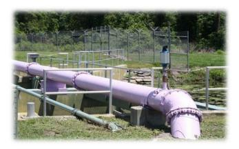
Another aspect of the RCID reuse system is the use of rapid infiltration basins (RIBs) for wet weather disposal and groundwater recharge. During wet weather periods (or when demands on the reuse distribution system are low) the RIBs are utilized for disposition of excess product water. Disposing excess reclaimed water in RIBs recharges the local aquifers.
