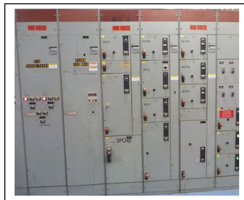
480V Motor Control Center “B”
