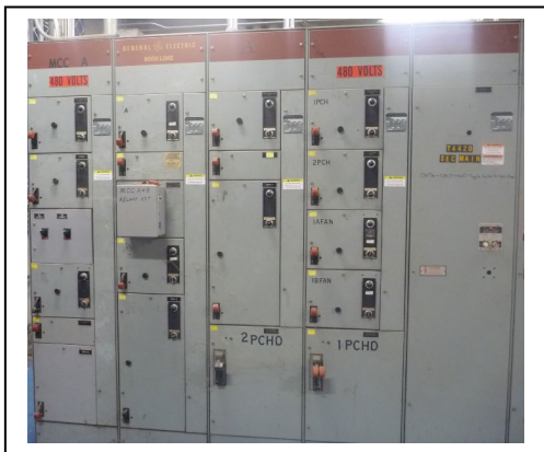
480V Motor Control Center “A”
